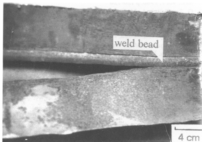
Fig. 1 Crack along the side of the weld
